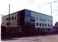
Norton's new headquarters provides key personnel with an excellent view of the company's operations - the South Canada Dock, weighbridge and baler area and the new shredder.
